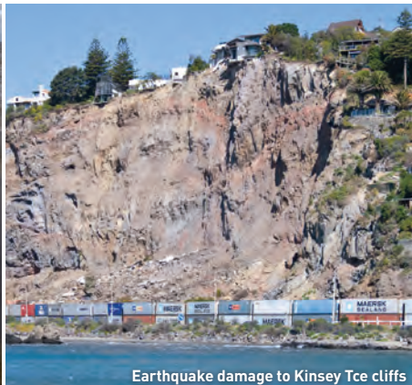
Earthquake damage to Kinsey Tce cliffs
