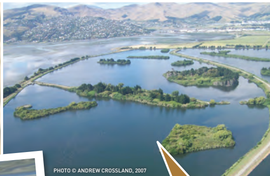
Wastewater treatment ponds from the air
