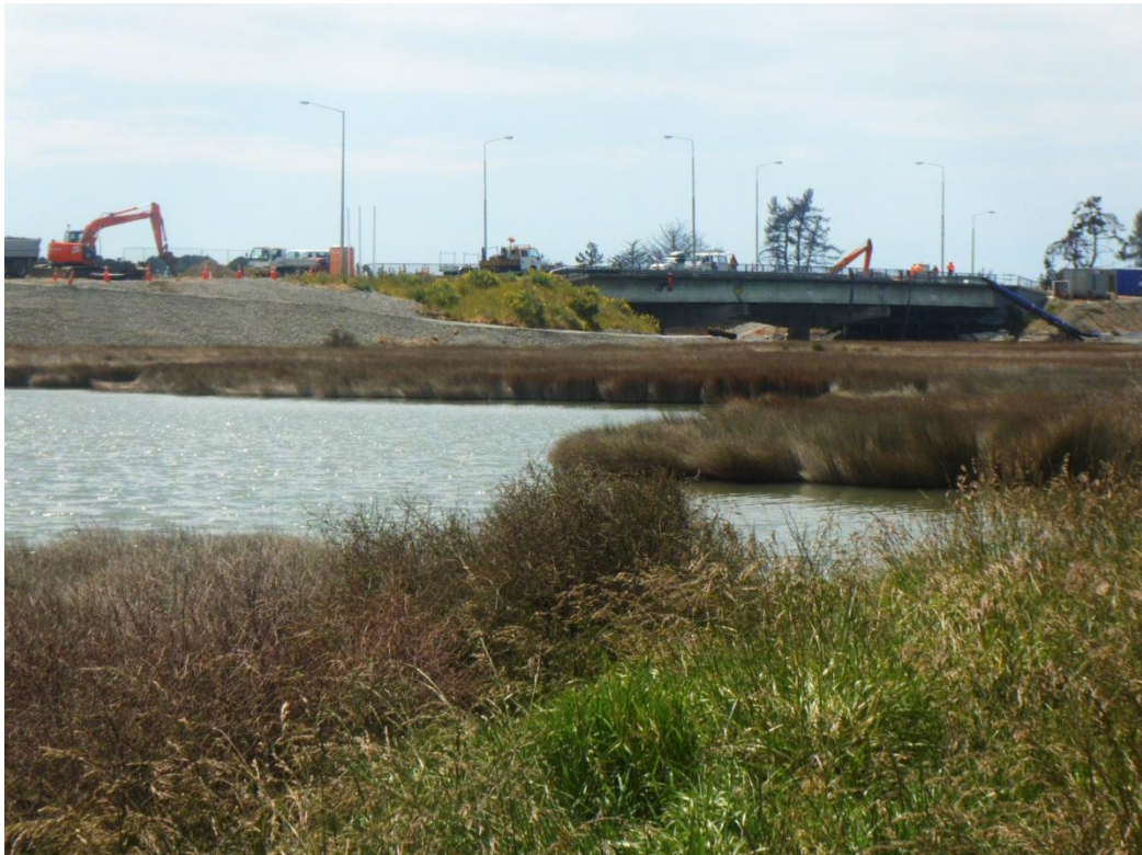
Figure 2: Bridge Street Bridge under repair
