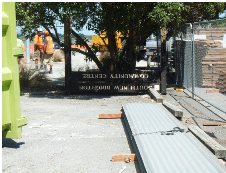
Figure 3: Demolition of South New Brighton Community Hall
